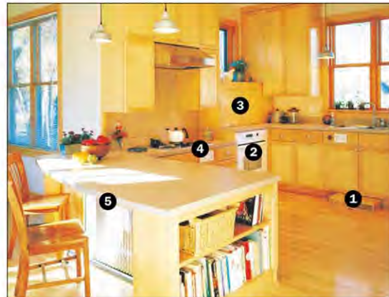
Accessible features aren't always obvious. 1. A pull-out step below the sink. 2. Easy-access oven. 3. Easy-to-reach appliance garage. 4. Easy-reach outlets and light switches at a reduced-height counter. 5. Roll-under countertop.
