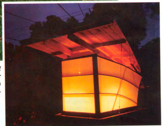
Warp factor two, Mr. Sulu! Bill Baxley and Vesa Loikas of Minneapolis designed and built this Dacron-polyester and cedar house; its roof channels rainwater into the carved drinking dish in the foreground. Photos by Bill Baxley.
